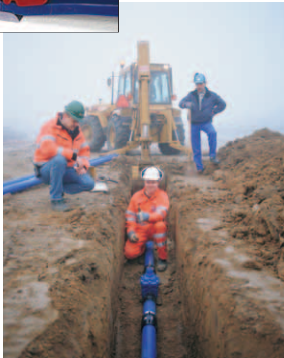
Installation of a PE-pipeline with AVK gate valves.
