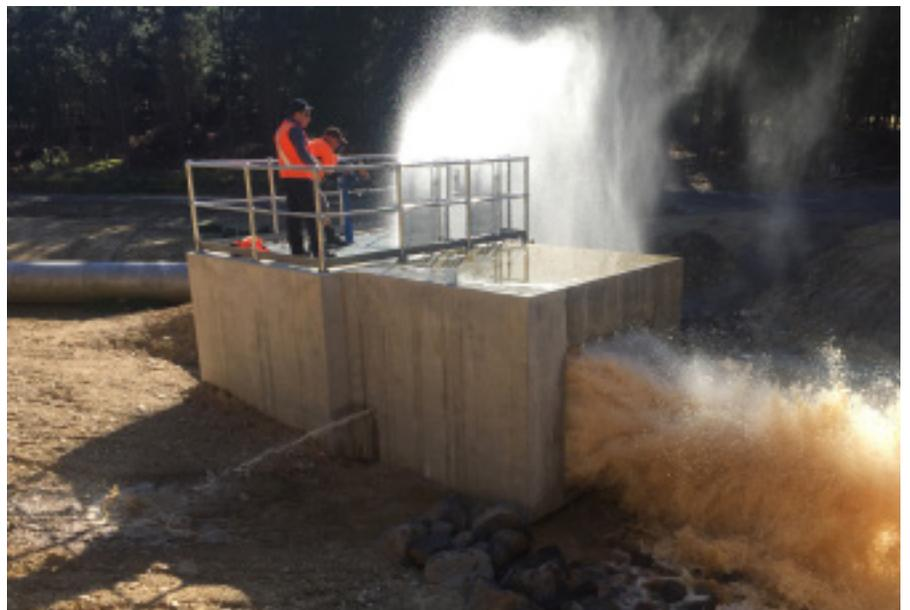
The initial enquiry for the White Swan Reservoir project commenced mid-year of 2015 when consultants from MWH Australia through the support from Louise Loughnan, Lead Engineer at MWH Global, first enquired about a DN600 discharge valve suitable for a new scour pipeline operating at 3.50 cumecs and a velocity of 7.91m/s.
