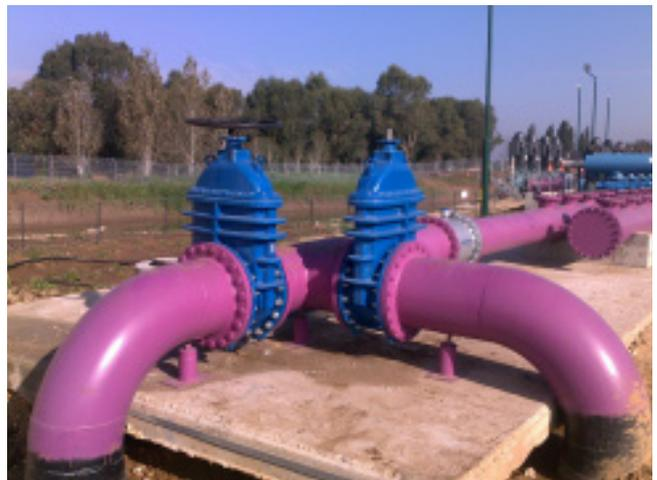
During a recent trip to Israel, I came across a different and more colourful installation of valves and pipes. They used the pink colour for installations with purified wastewater which is used for watering crops.
