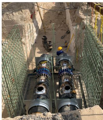
Products delivered to the project include Desponia butterfly valves from InterApp, manual and motorized from DN200 to DN600, PN16, 164 pieces in total. From AVK Anhui, series 756 motorized butterfly valves DN1600, 6 pieces.
