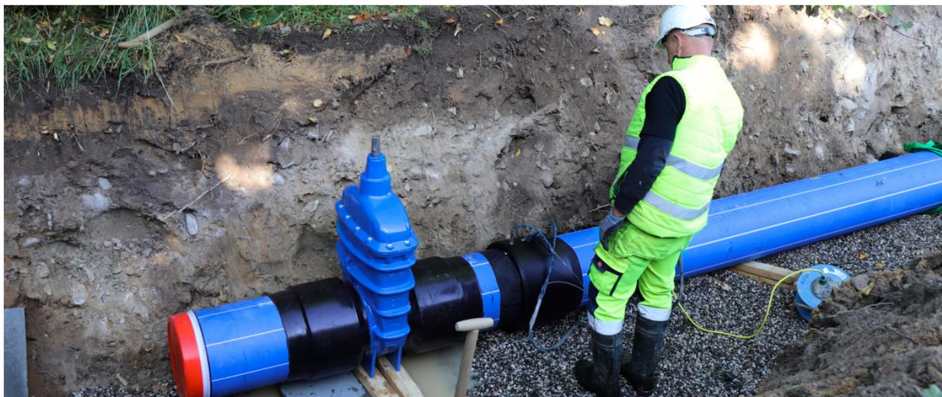
A fully welded PE pipe system offers a lot of benefits such as reduced risk of leakage, ease of installation and a high durability. We have recently launched gate valves with PE ends in four new sizes with outside pipe diameters of 450, 500, 560 and 630 mm, so with AVK gate valves with pre-mounted PE pipe ends you can now design a fully welded pipe system up to 630 mm.
