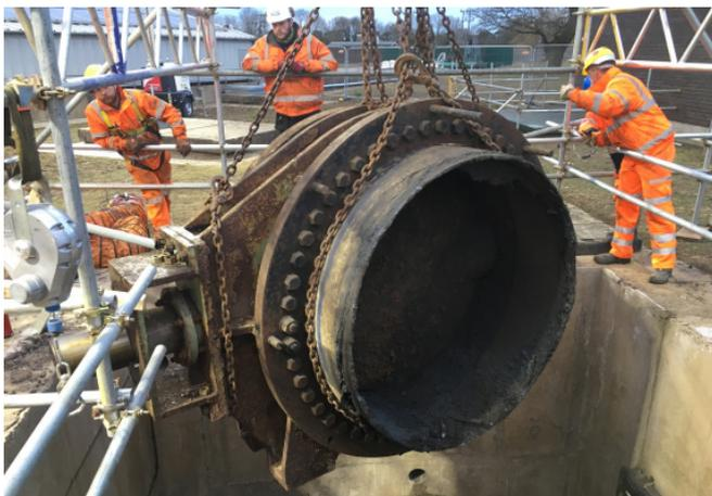
"The butterfly valve is a critical element of the pumping station's infrastructure and we undertook a detailed engineering survey of the site before removing the valve. However, as any
